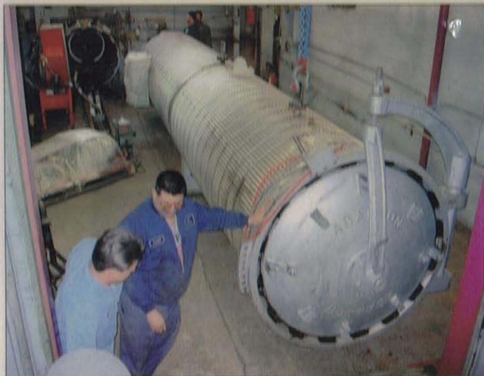
Plant Manager Glenn Kuras (left) and Arnold Amar, who heads up the maintenance department at Passaic Rubber Co.'s facility in Wayne, N.J., discuss the workings of the company's new large diameter electric autoclave as it's being rigged up.
